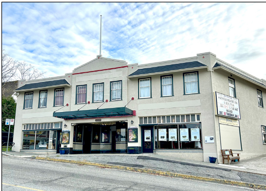
Restorations to the Historic Patricia Theatre are nearing completion
